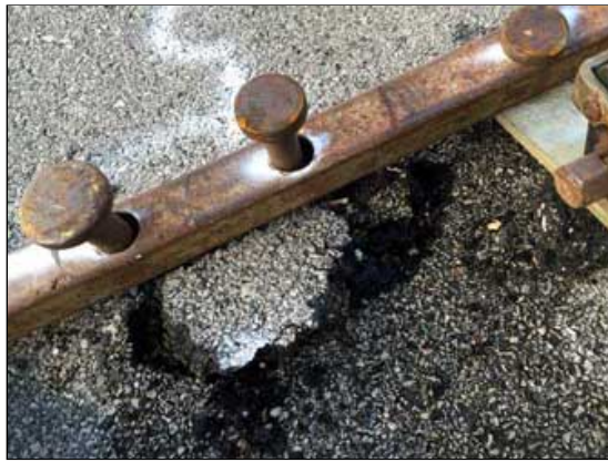
AFTER PHOTOS - ASPHALT PATCH APPLIED
