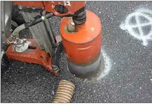
6-IN CORE BEING DRILLED IN ASPHALT PAVEMENT
