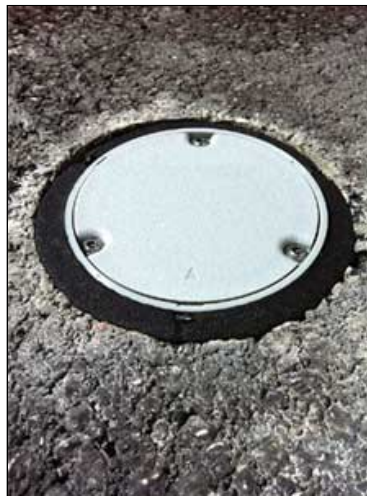
HOLE CAP INSTALLED FOR REUSING ANCHOR
