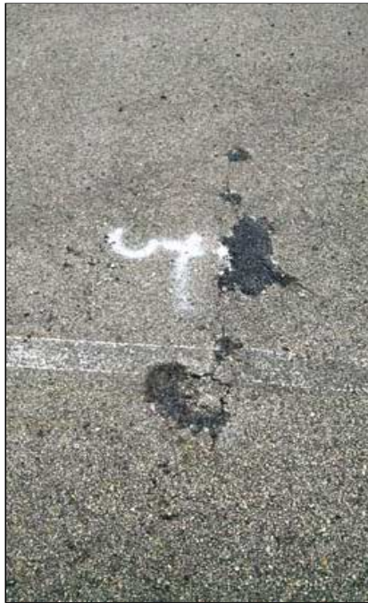
AFTER PHOTOS - ASPHALT PATCH APPLIED
